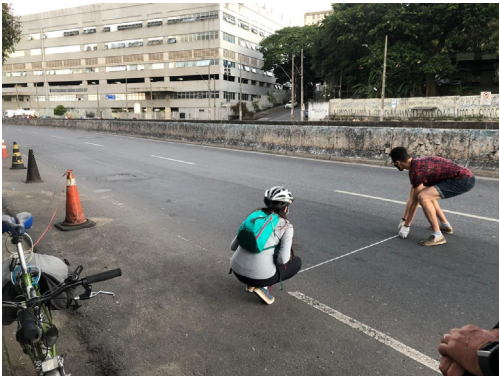
Figure 6. Creation of temporary bike lanes in the city of Belo Horizonte, Brazil. Source: Belo Horizonte Transport Authority
