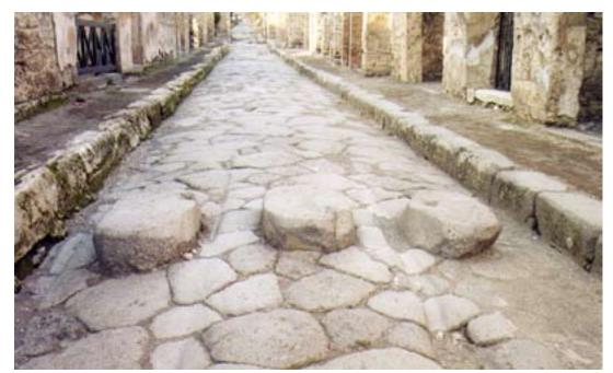
Fig. 28 A vehicle restriction device that was employed in ancient Pompeii. Photo by Lloyd Wright
